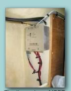
The three phase MPPT charger/regulator from Blue Sky mounted in the cockpit locker adjacent to where the water heater used to be.
