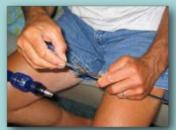
Fitting the cone over the core wires during the install of a Hayn Hi-Mod backstay insulator.
