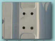
Over-drilling and filling the tack plate holes with epoxy, which are then under-drilled for the through bolts, first step in converting to a cutter.
