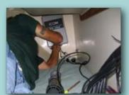
Installing the ICOM AT-140 automatic antenna tuner at the aft end of the quarter berth (not a bunk that will be occupied, obviously).
