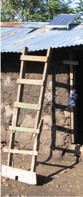
After we install the solar panel, maybe we should fix the ladder.
