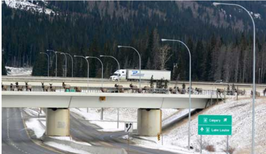
Figure 4. Road impacts are so severe in some places that special highway overpasses or tunnels have to be built to allow safe passage of animals within their normal range. (Image from http://www.huntingvt.com/wildlife-pictures.htm : downloaded 9/13/2010)
