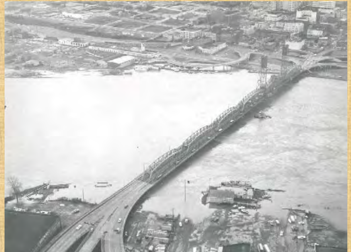
At Hawthorne Bridge
