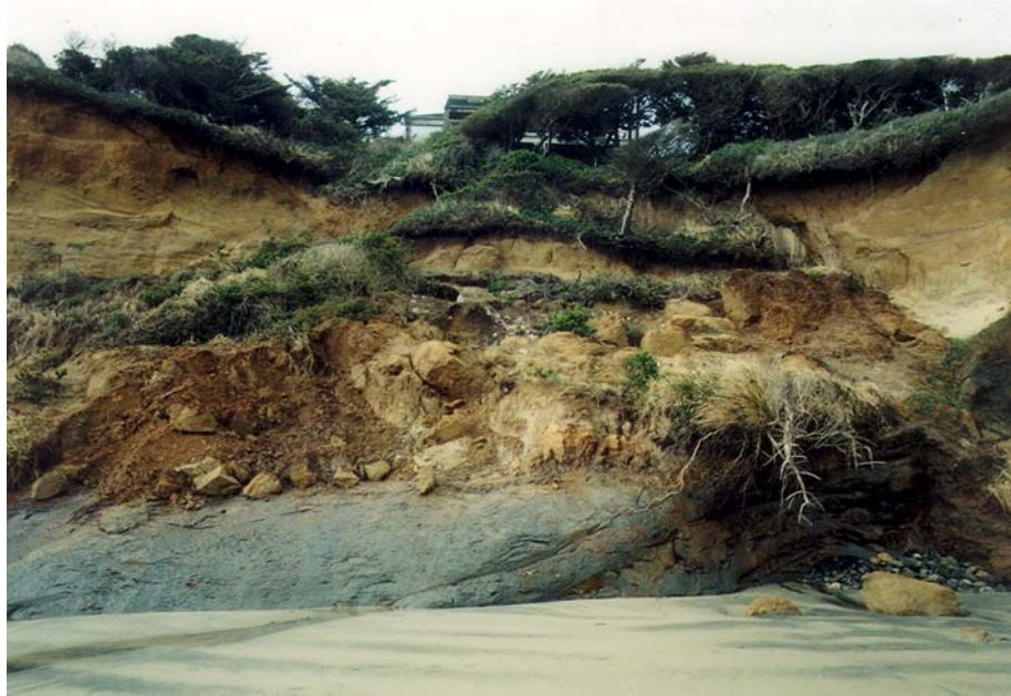
Figure 72: A slump slope failure in the Newport dune sheet. The bedrock acts as an aquitard allowing the ground water flow to concentrate at the contact between the paleodune deposits and the bedrock. The concentration of ground water leaches out the cement from the dune sheet deposits weakening the basal layer.
