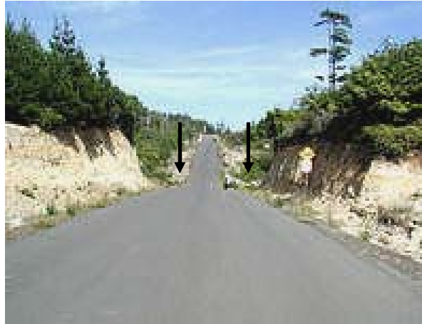
Figure 24: Road cut heading east from Highway 101 through paleodune deposits. The area on both sides of the road is zoned for residential development. The dip in the road (shown by arrows) is an interdunal stream running north to south.
