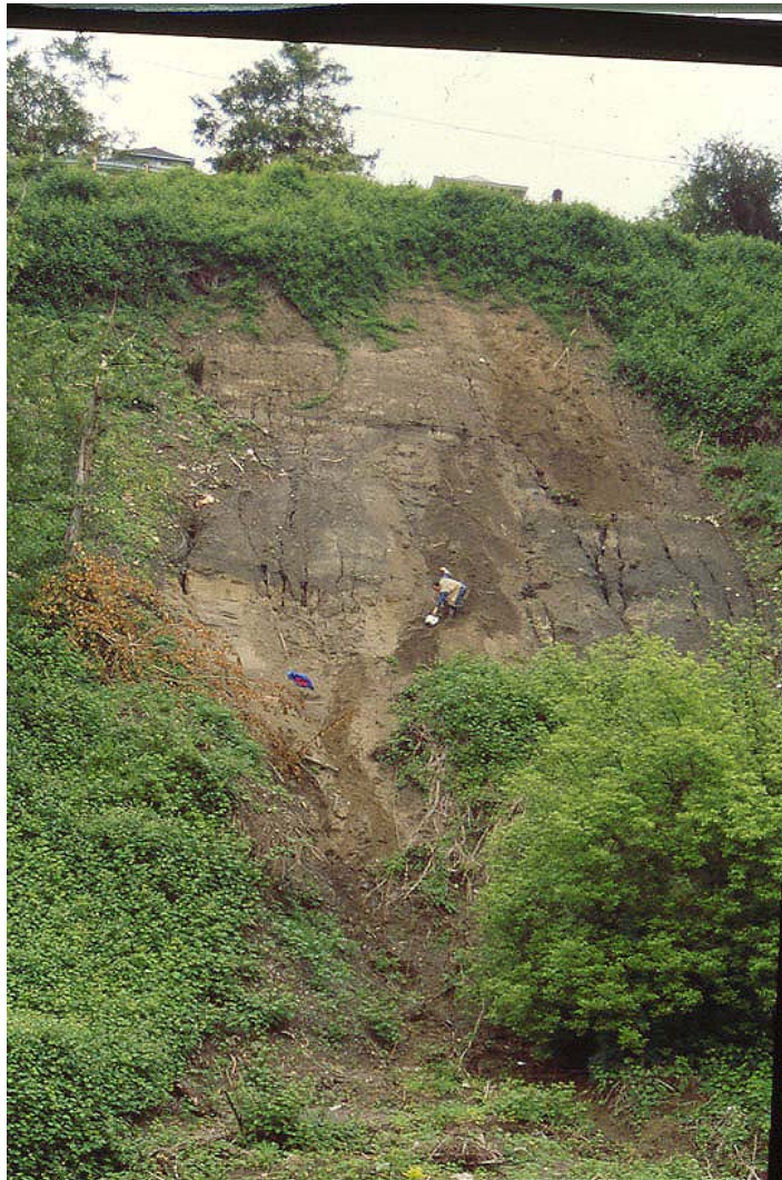
Figure 10. Greeley Avenue site, north Portland (note geologist in center for scale).
