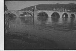
129098 Neckar River Bridge, Heidelberg.
