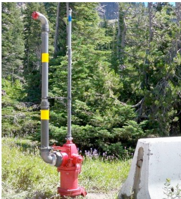
+ View full size Scott Freeman Lt. John Creel of the Hoodland Fire Department in Welches patented a hydrant snorkel design. This is one being tested at Crater Lake National Park.
