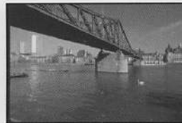
129090 Main River Bridge, Frankfurt.
