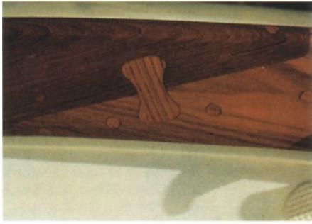
Teak "Butterfly" inserts lock together caprail joint so that they will never separate
