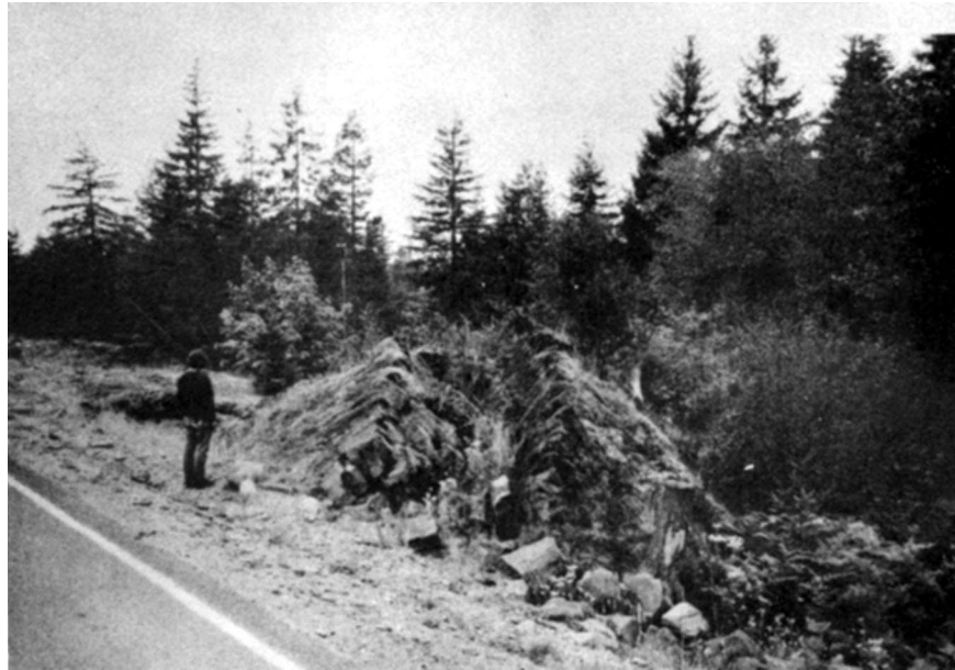
Figure 4. Pressure ridge with medial crack, mile 52.5.
