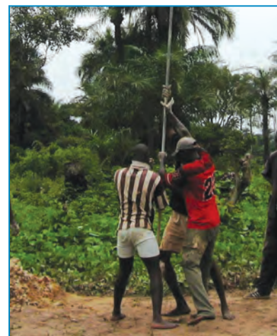
Hand Auger 15-25 meters, depending on the geology.
