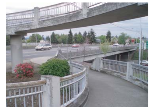
~11' 7" vertical clearance between bridge and access ramp below
