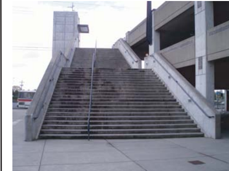
Stairway at bridge's north end
