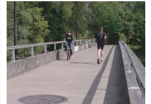
Bridge cross-section includes a 12' width (railings and walls are flush with one another)
