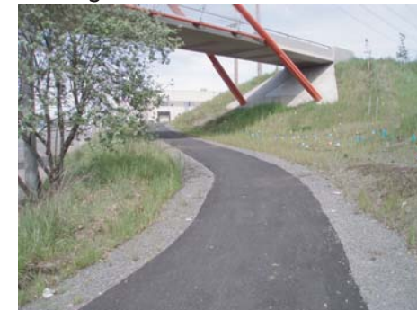
Access ramp connecting bridge with SE McLoughlin Blvd.
