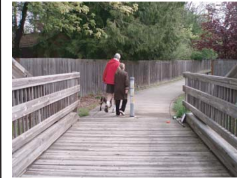
Bollards placed at the bridge's center provide sufficient clearance for passing bicyclists, wheelchairs and other users
