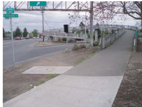
No physical or other elements exist to discourage at-grade crossings of the I-5 entrance ramp
