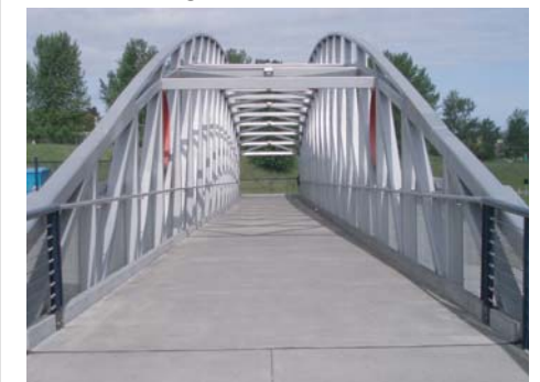
Bridge cross-section includes a 12' rail-to-rail width
