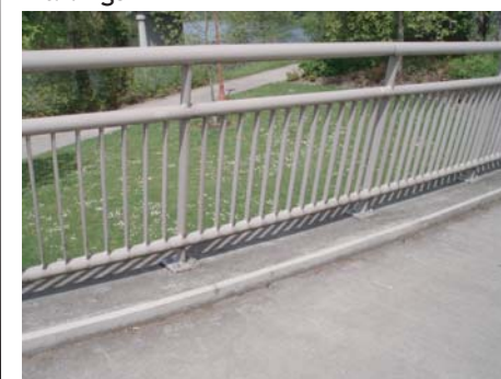
Railing style on bridge structure and north access ramp
