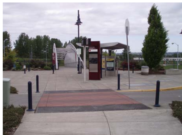
Figure 11 – Raised crosswalk near the I-205 at Parkrose Transit Center Bridge
