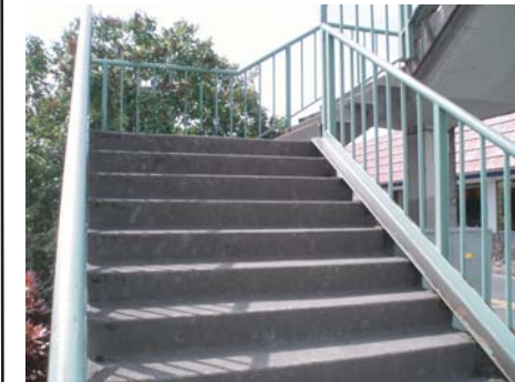
Stairway with landings and "bike gutter"
