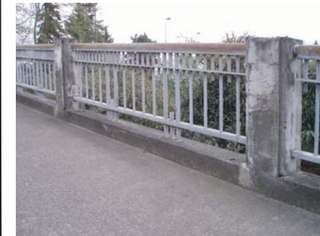
Railing style on access ramps and bridge
