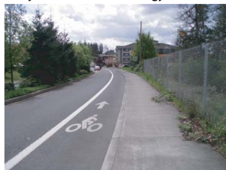
Bicycle lanes and sidewalks on SW Bangy Rd.
