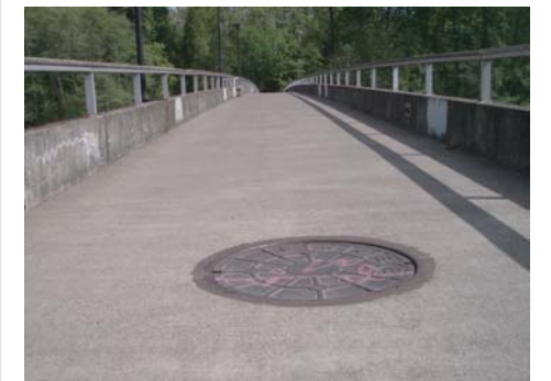
Manhole cover on bridge deck
