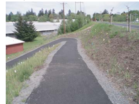
Switchback on east access ramp
