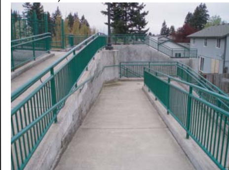
North access ramp
