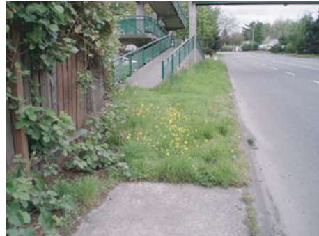
Gap between bridge access ramp and sidewalk on N. Columbia Blvd.
