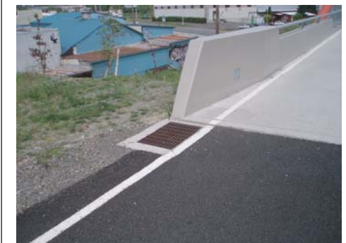
Drainage grates placed outside the bicycle/pedestrian travelway
