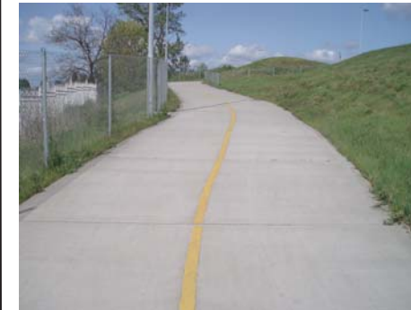
North access ramp
