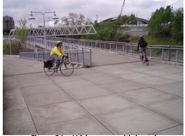
Figure 21 – Wide ramps with broad switchbacks on the Eastbank Esplanade-Rose Quarter Connector
