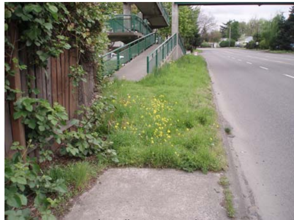
Figure 10 – Sidewalk gap complicates access to the N Columbia Blvd. at Midway Ave. Bridge
