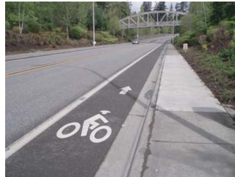
Bicycle lanes and sidewalks on Cedar Hills Blvd.
