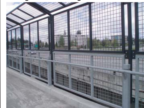
Railing style on bridge structure
