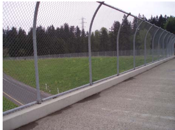
Figure 31 – Fencing on the I-5 near Main St. Bridge is about 10' 5" tall
