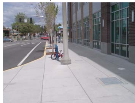
Bicycle lane without transition ramp from sidewalk/cycletrack (north side of bridge)
