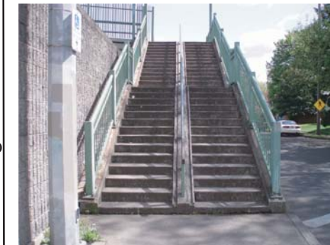
Stairway with "bike gutter" on bridge's south end
