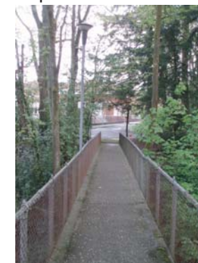
Light pole on bridge structure
