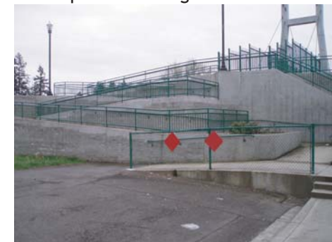
Narrow access ramp with multiple switchbacks complicates bicycle access on the bridge's north end
