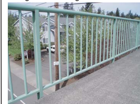
Railing style on stairways and bridge
