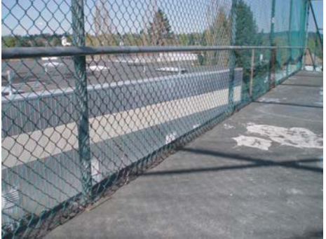
Railing style on stairways and bridge
