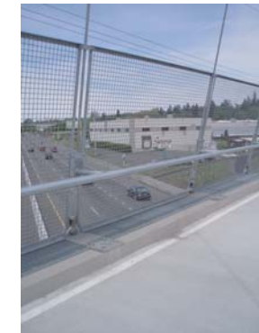
Railing style on bridge structure
