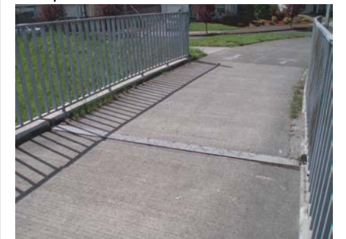
Expansion joint gap at bridge's west end
