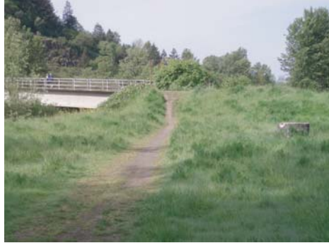
Informal path at bridge's north end
