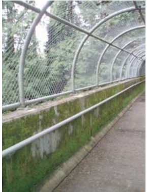
Railing style on bridge
