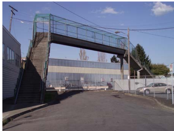
Figure 6 – Stairways are the only access provision at the SE Brooklyn St. at Union Pacific Railroad Bridge
