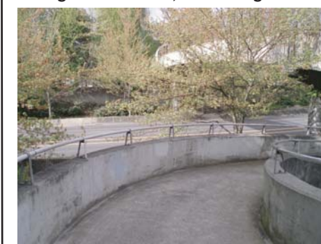
South access ramp
