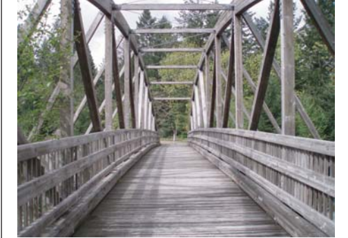
Bridge cross-section includes a 10' curb-to-curb width, plus 3.5" of "shy distance" on each side
