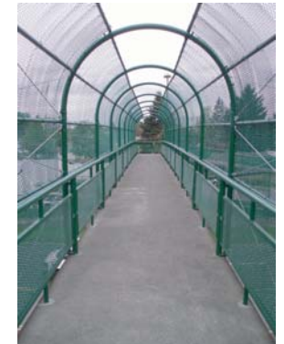
Bridge cross-section includes a 6' rail-to-rail width
