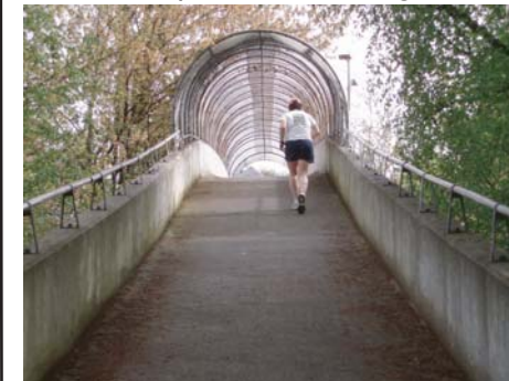
Access ramp slope is relatively steep immediately near the bridge structure
