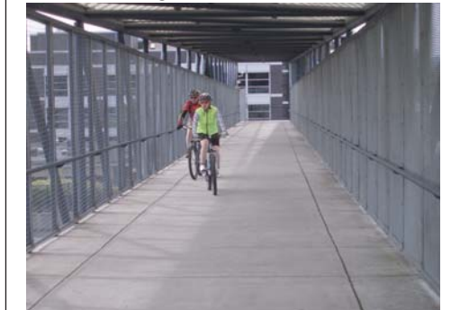
Bridge cross-section includes an 11' 1" rail-to-rail width
