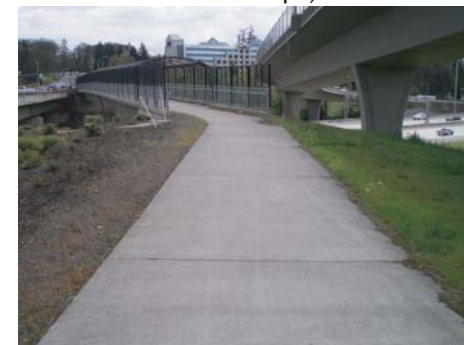
Bridge and path are at roughly the same elevation, eliminating the need for stairways or circuitous access ramps
