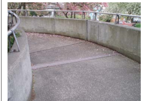
Drainage grates are flush with the pavement, thereby easing travel for "wheel" users
