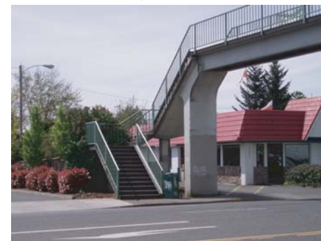
Stairway oriented perpendicular to SE Division St.
