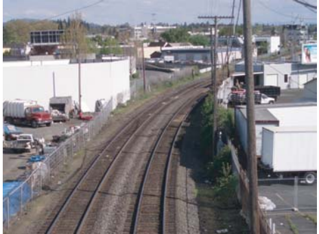
Fencing on both sides of the railroad preclude at-grade crossings
