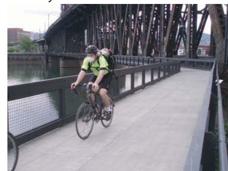
Steel Bridge Bikeway/Walkway
