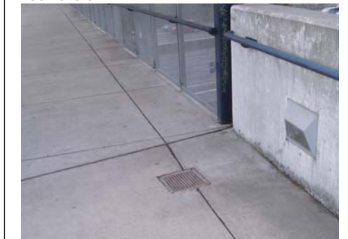
Drainage grate at bridge's north end
