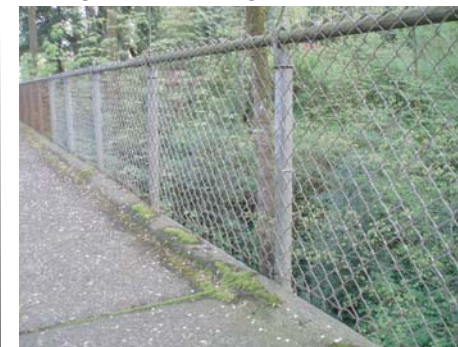
Railing style on bridge
