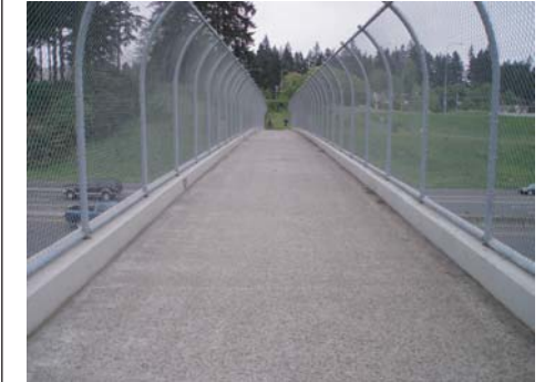
12' curb-to-curb width on bridge structure
