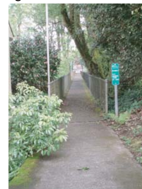
Bridge and surrounding streets are at roughly the same elevation, therefore requiring no stairways or circuitous access ramps
