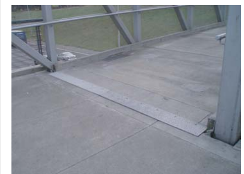
Expansion joint "lip" at bridge's west end
