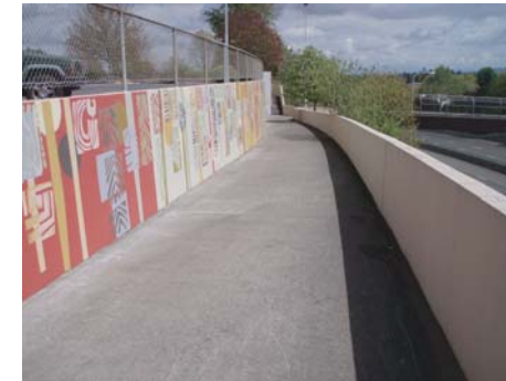
North access ramp
