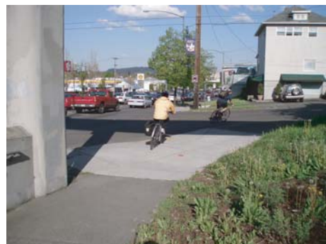
Curb ramps provided where bridge access ramps meet the surrounding street system
