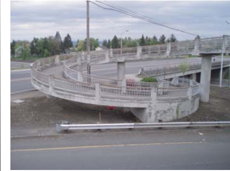
East access ramp
