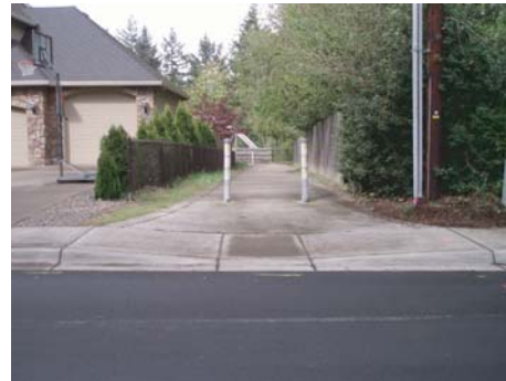
Accessway connecting the bridge with NW 112th Ave. provides curb ramps for easy bicyclist transitions to/from the street
