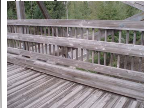
Railings on bridge structure
