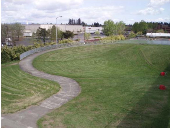
Figure 17 – Curvilinear access path near the I-205 at SE Main St. Bridge
