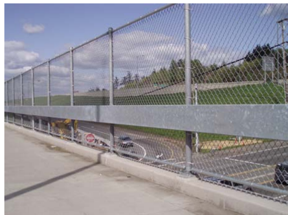
Figure 32 – Bicycle "rub rail" on the SE Powell Blvd. at I-205 Bridge
