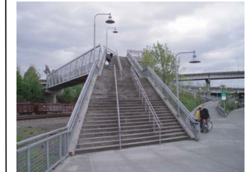
Stairway with landing on bridge's west end
