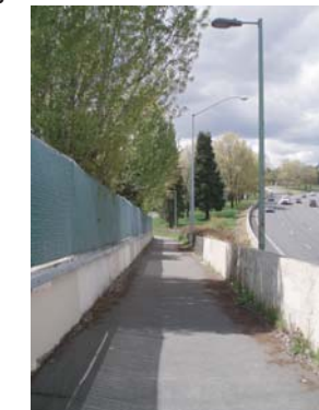
Lighting on south access ramp
