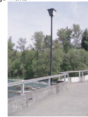
Overhead lighting on bridge
