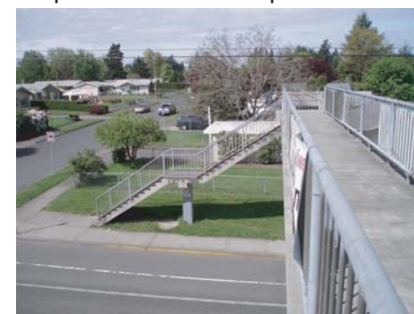
At each bridge end, stairways are oriented in one direction of travel only, which may not be useful to pedestrians wishing to travel in the opposite direction
