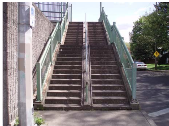
Figure 22 – Stairways near the I-84 at Hollywood Transit Center Bridge include “bike gutters”
