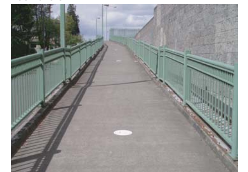
The bridge and access ramps benefit from relatively good pavement conditions
