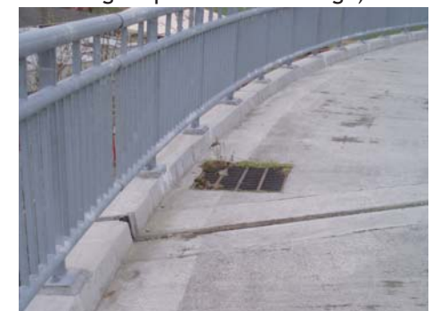
Drainage grate and expansion joint on bridge structure
