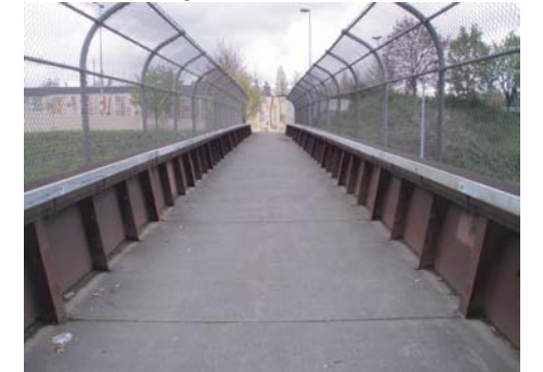
Bridge cross-section includes an 11' rail-to-rail width
