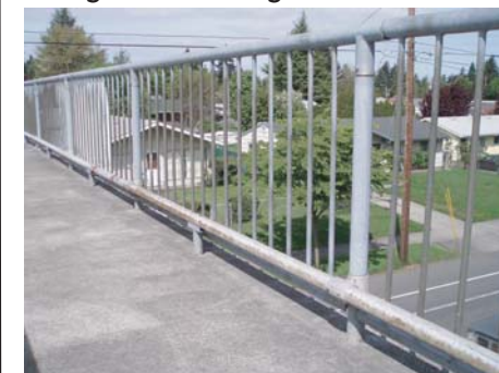
Railing style on stairways and bridge
