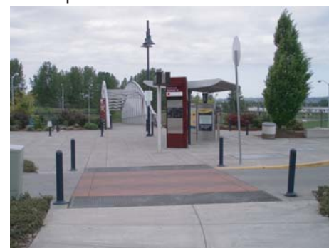
Raised crosswalk at bridge's east end
