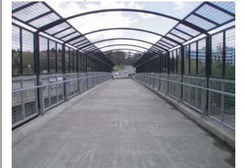
Bridge cross-section includes a 14' rail-to-rail width
