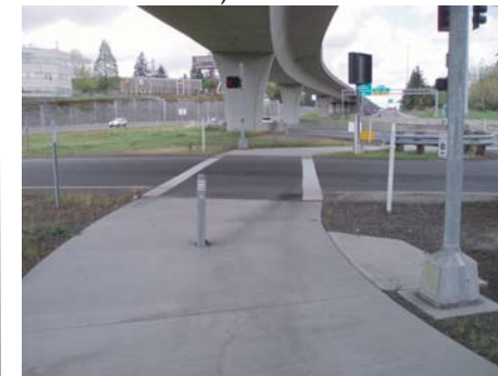
Center bollard present where shared use path meets intersection west of the bridge
