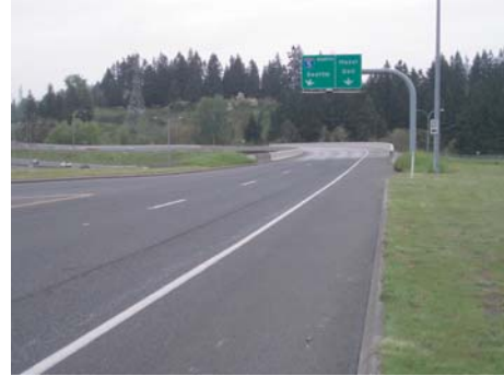
The nearest alternative crossing (I-5 at Main St.) lacks sidewalks
