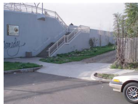
Driveway apron on the bridge's east end facilitates easy bicycle transitions to/from the street
