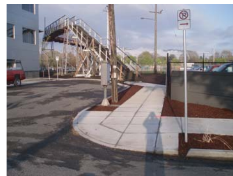
Sidewalk and curb ramp in good condition near east stairway
