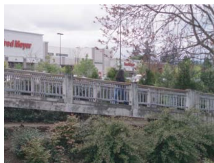
Commercial area near bridge
