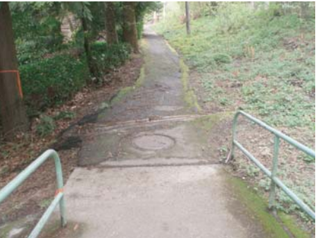
Pedestrian path on the bridge's north end
