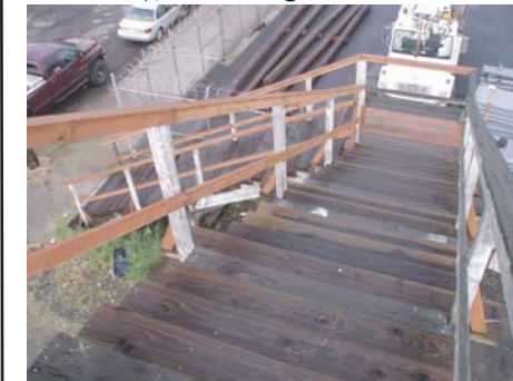
Railing style on stairways
