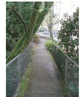
Encroaching vegetation on sidewalk near bridge's west end
