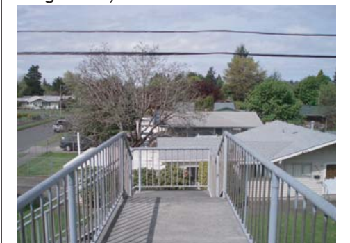
Low-hanging electrical wires above bridge
