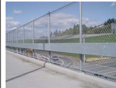
Bridge railing also serves as a bicycle "handlebar guard"
