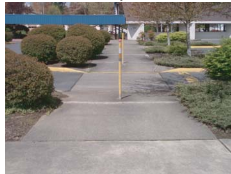
Sidewalk connecting north access ramp with Barbur Transit Center
