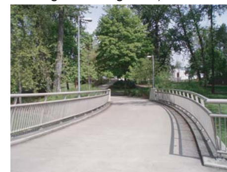
North access ramp
