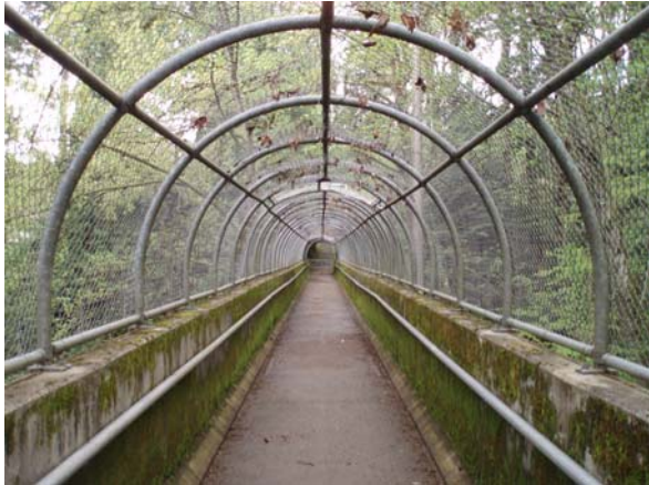
Figure 24 – A relatively low vertical clearance creates the perception of isolation on the Trillium Cr. Bridge
