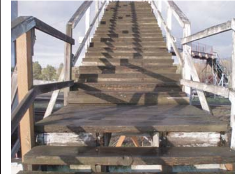
Wooden stairway with landings
