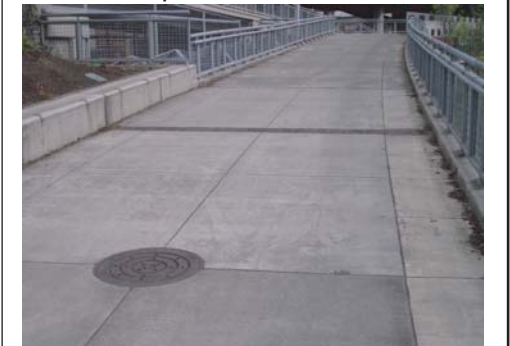
Drainage grates and manhole covers are flush with the pavement
