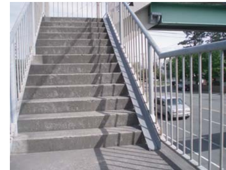
Stairway with landings and "bike gutter"
