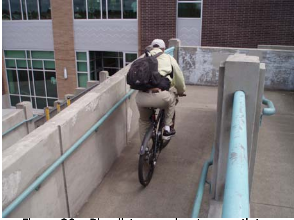
Figure 20 – Bicyclist preparing to negotiate a narrow switchback turn approaching the I-84 at Hollywood Transit Center Bridge
