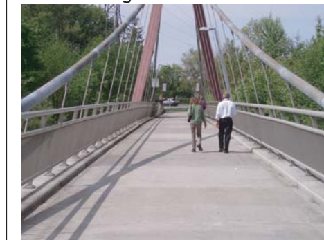
Bridge cross-section includes a 14' width (curbs and railings are flush with one another)
