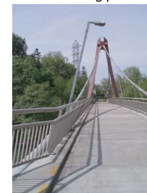
Lighting on bridge structure
