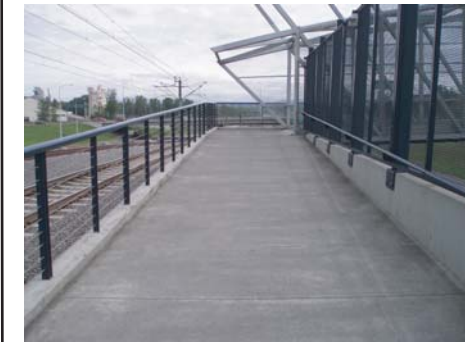
West access ramp
