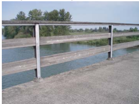
Railing style on bridge structure
