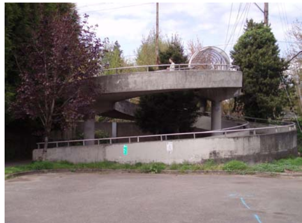
Figure 19 – Spiral ramp on the N Going St. at Concord Ave. Bridge
