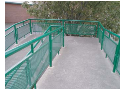
Access ramp with level landings
