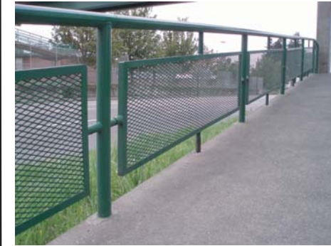
Railing style on access ramps and bridge
