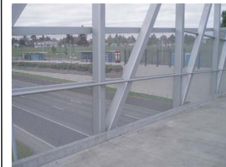
The bridge structure includes 42" high railings on both sides
