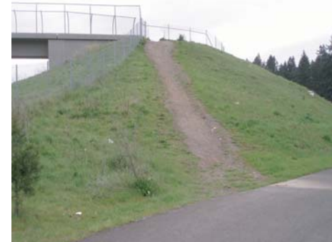
Informal path created by bridge users to reduce out-of-direction travel
