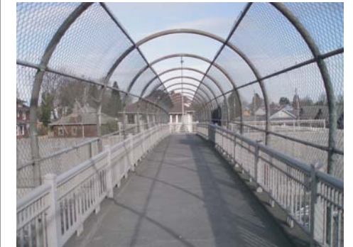
Bridge cross-section includes an 8' curb-to-curb width
