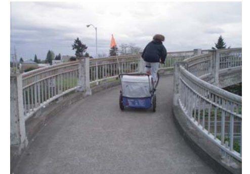
Bridge cross-section includes an 8' curb-to-curb width
