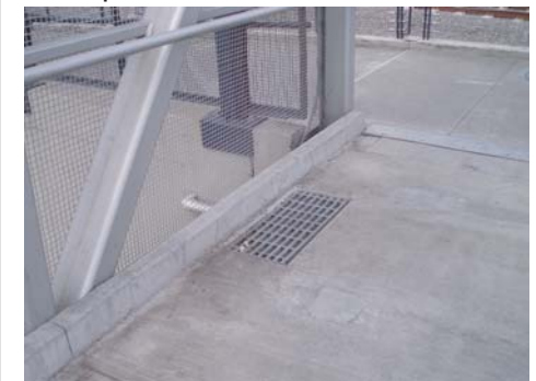
Drainage grate at bridge's west end
