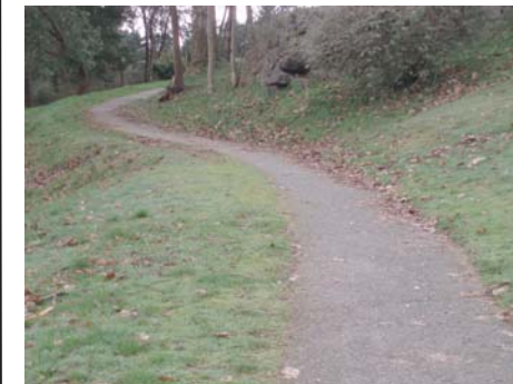
East access path
