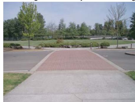
Raised crosswalk with pavement texturing on Millrace Dr. immediately south of the bridge
