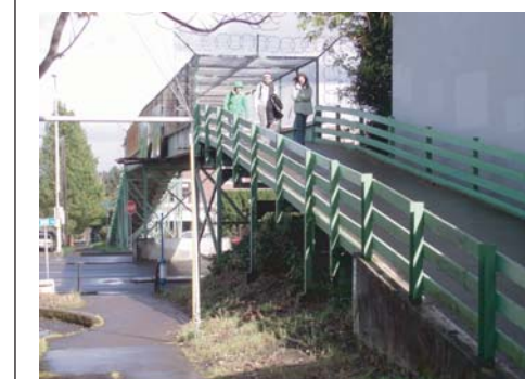
The linear ramps provide direct access between the bridge and points farther east and west, but require additional travel for users accessing TriMet bus stops directly under the bridge
