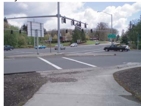
Pedestrian infrastructure present on SW Kruse Way at Bangy Rd., immediately east of the bridge
