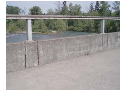
Railing style on bridge structure
