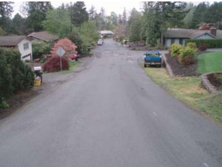
Sidewalks lacking on SW Boundary St. north of the bridge
