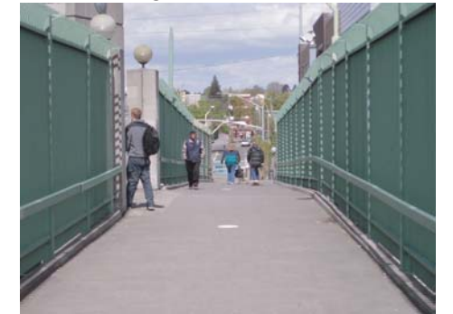
Bridge cross-section includes an 11' 6" width (curbs and railings are flush with one another)
