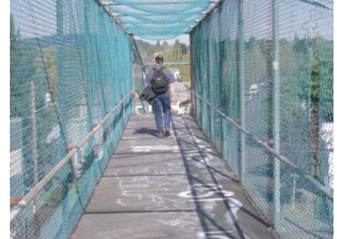
Bridge cross-section includes a 5' 7" rail-to-rail width
