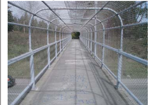
Bridge cross-section includes a 7' 6" rail-to-rail width and a 7' 6" vertical clearance
