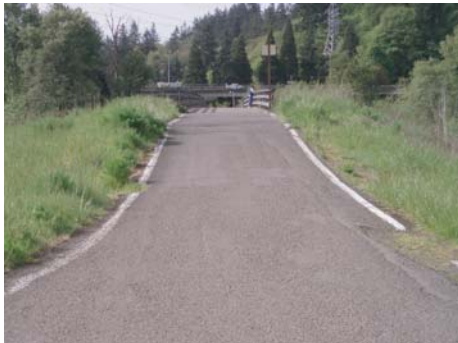
The north access path includes a short but steep grade, which can pose difficulties for wheelchairs and other users
