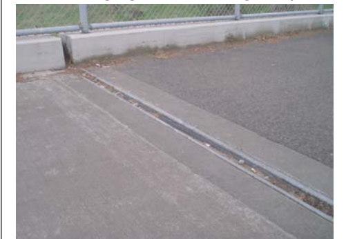
Expansion joint gap at west end of bridge structure
