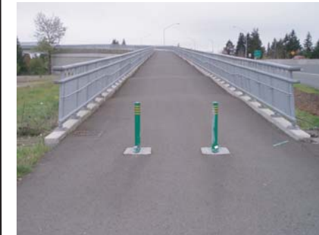
Twin bollards near east end of bridge
