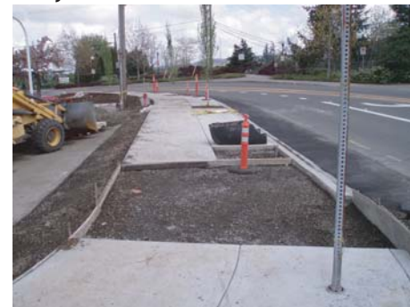
Sidewalk under construction on SW Butner Rd.
