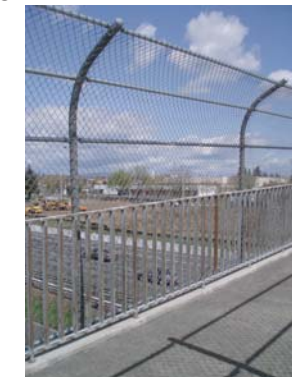
Fence and railing on bridge structure
