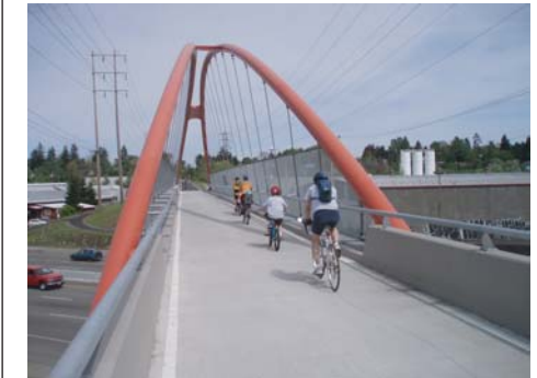
Bridge cross-section includes a 12' width (curbs and railings are flush with one another)
