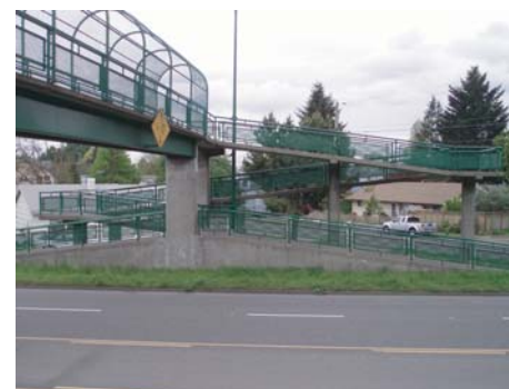
Bridge users must negotiate through several switchbacks on both ends of the structure
