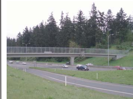
The only source of lighting is provided by surrounding light poles on I-5
