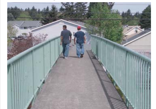
Bridge cross-section includes a 5' 11" rail-to-rail width
