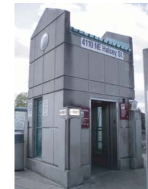
Elevator providing access between bridge and MAX station below
