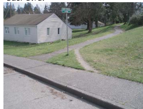
Curb ramps lacking where access paths meet surrounding streets
