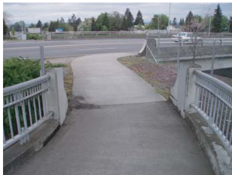
Transition between sidewalk and bridge access ramp
