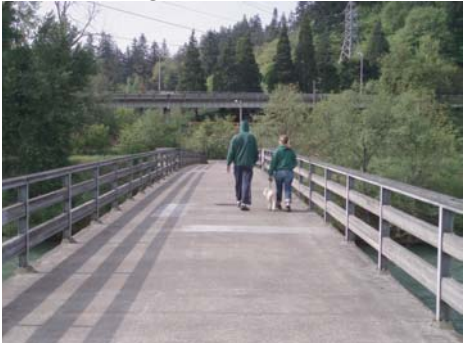
Bridge cross-section includes a 13' rail-to-rail width
