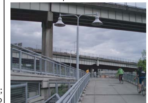
Lighting on west access ramp
