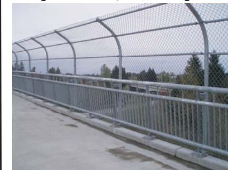
Railing and fence on bridge structure
