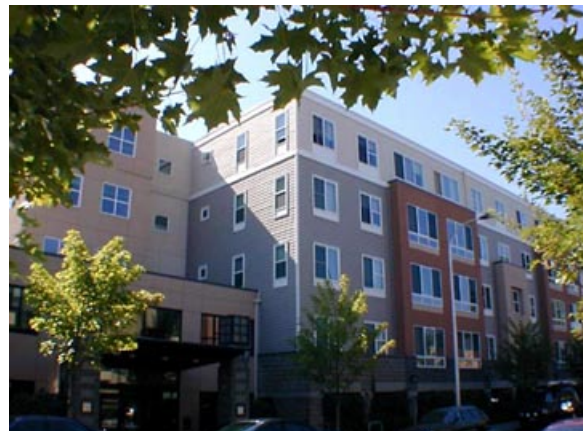
Photo of Site 4
