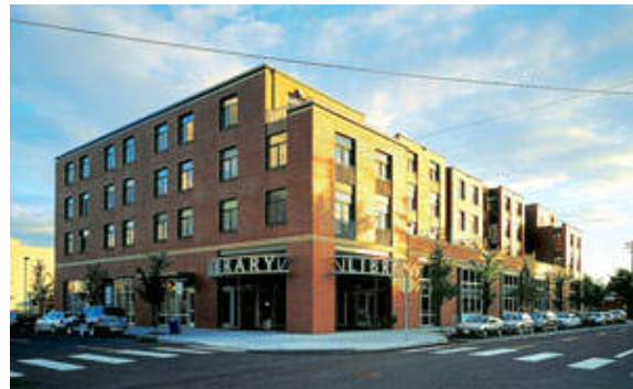
Photo of Site 2
