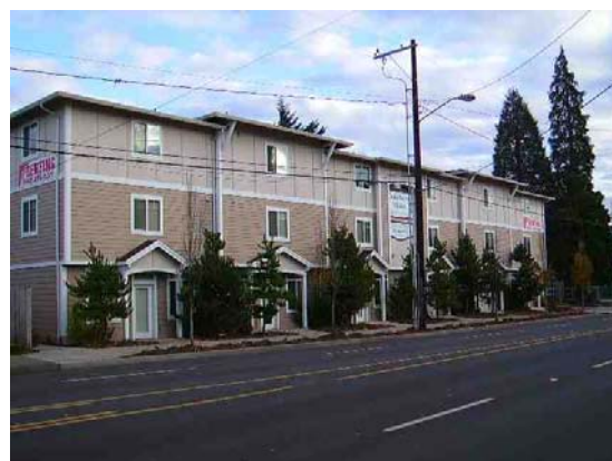
Photo of Site 3
