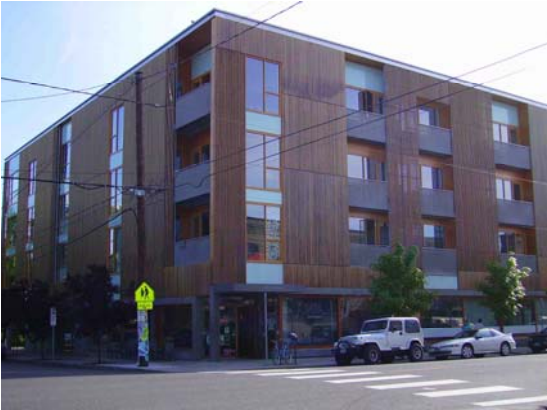
Photo of Site 5
