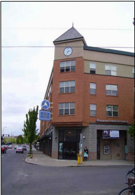
Photo of Site 1
