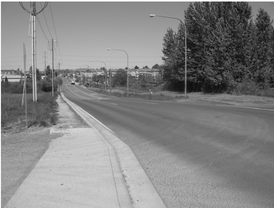
Figure 16: End of Sidewalk between Arbor Station and MAX Station
