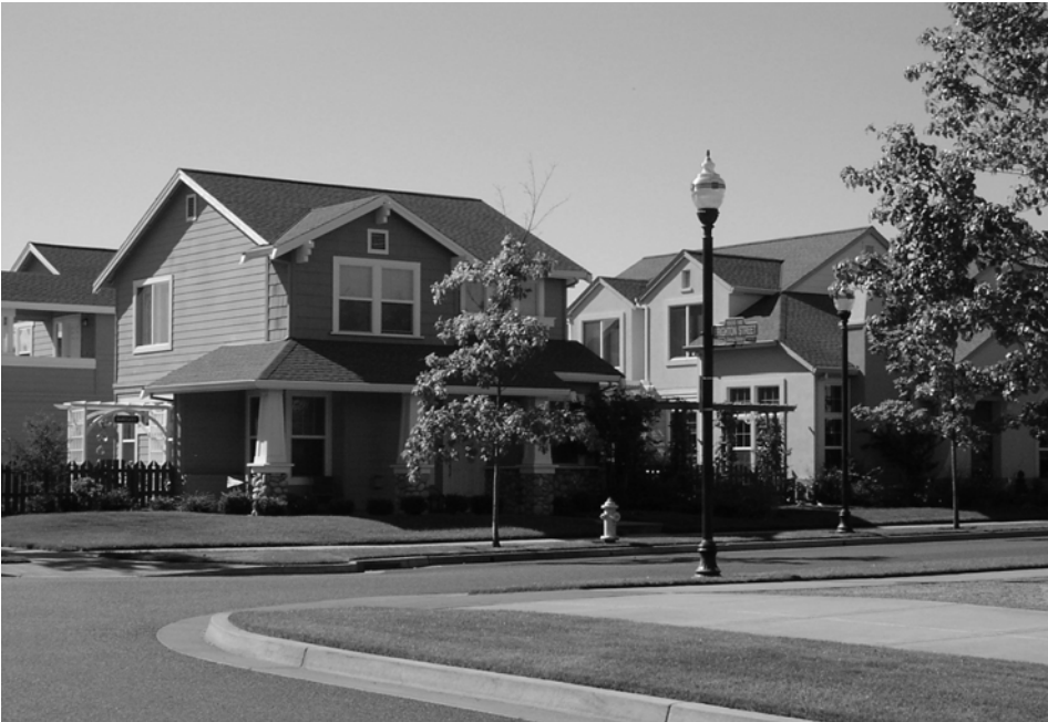
Figure 6: Original Orenco Station - Single Family Homes
