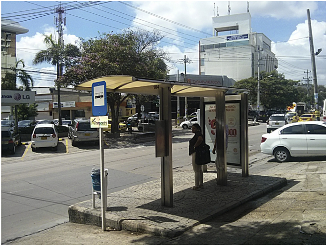
Fig. 4. Transmetro Barranquilla bus stop. Source: Authors.
