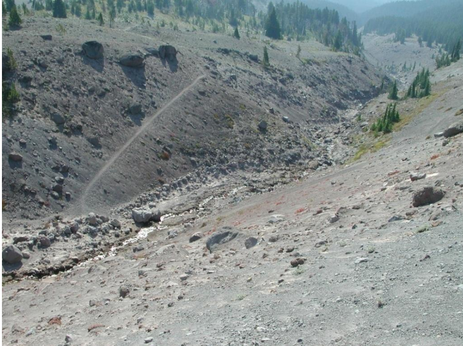
Figure 37. Salmon River boulder levees
