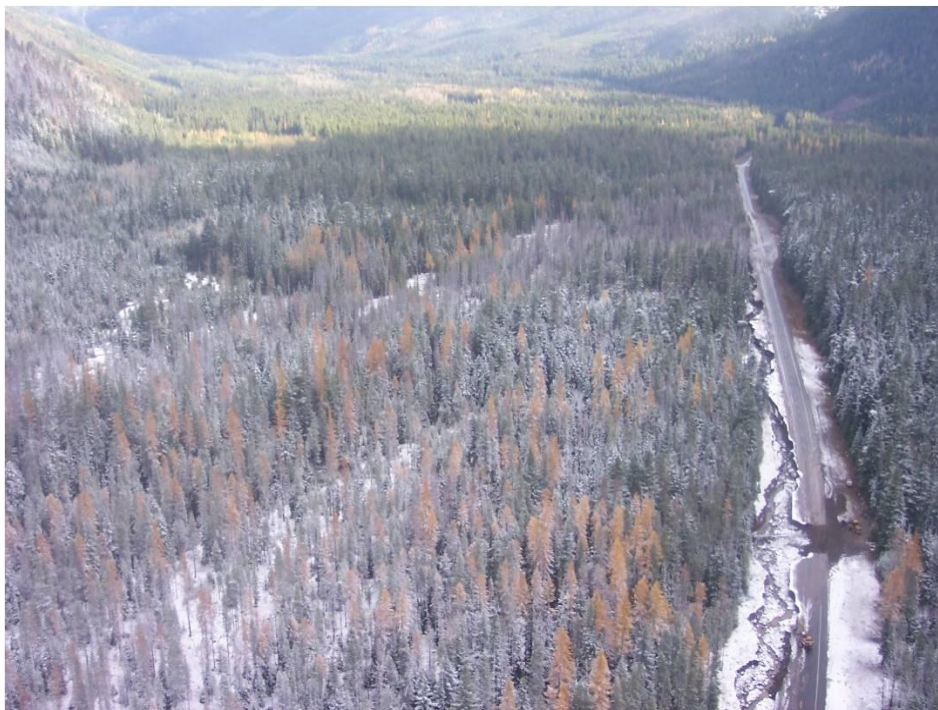
Figure 30. Highway 35 damage east of Hood River Bridge (photo courtesy of ODOT)
