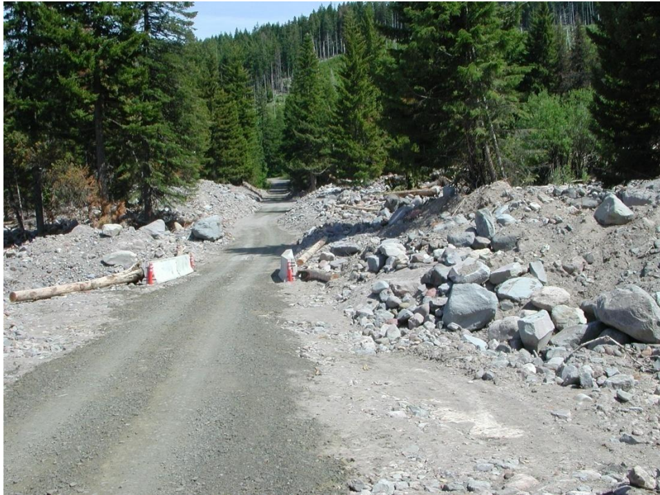
Figure 8. Laurance Lake Road at Eliot Creek crossing
