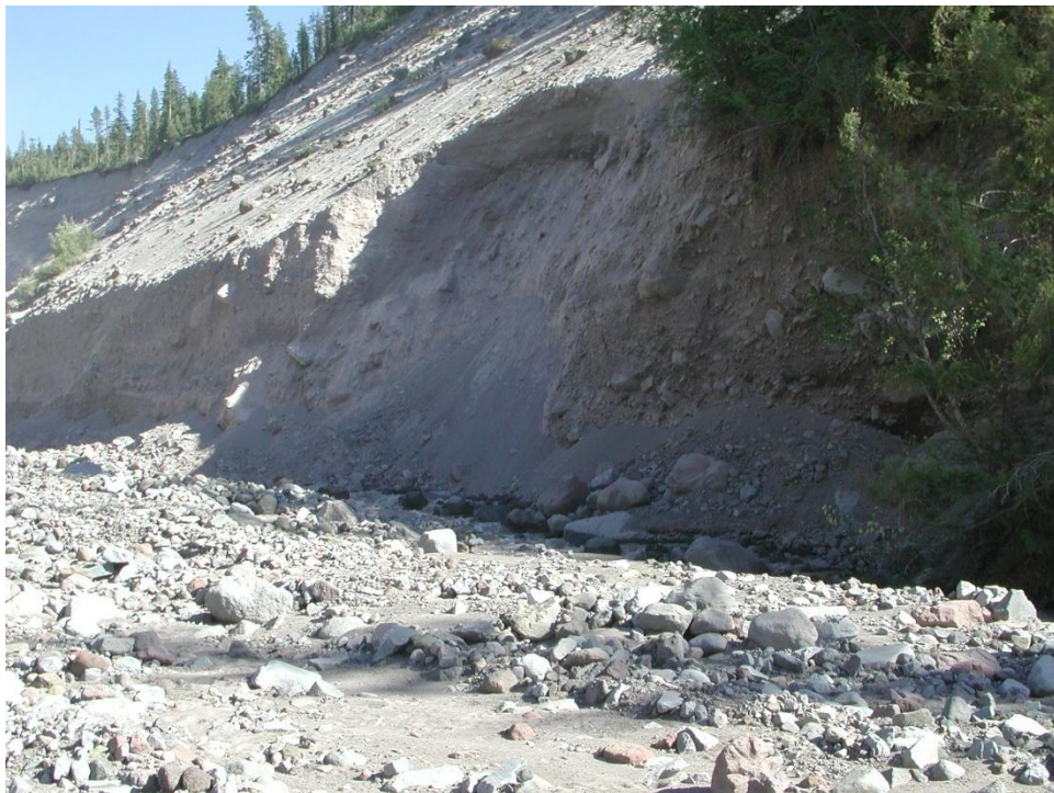
Figure 20. Landslide along steep canyon wall upstream from the Timberline Trail
