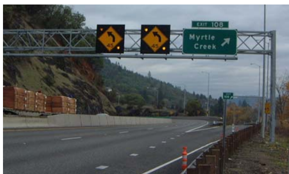
Figure 8: Northbound, Before Treatment
