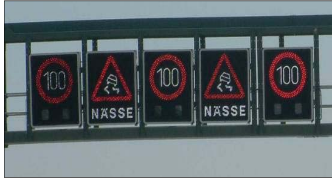
Figure 1 - Sample VSL gantry
