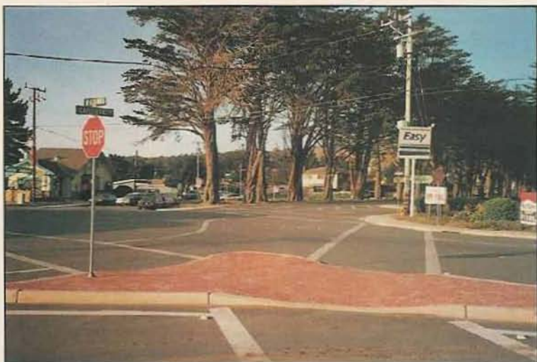
Avenue Alhambra, after rehabilitation. The Alhambra project offered project planners the opportunity to improve virtually every element of the aging and scenic roadway. As this photograph shows, the system of intersections was vastly clarified during rehabilitation.
