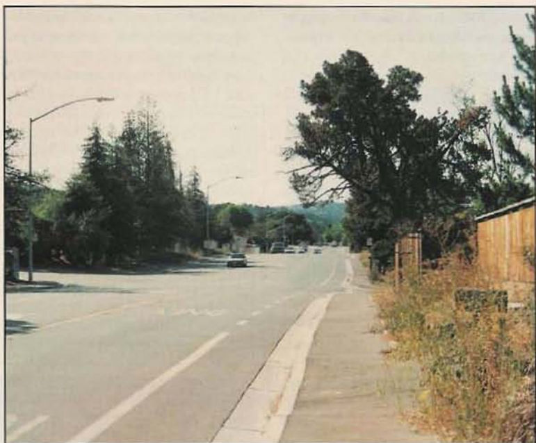
Alameda de las Pulgas after renovation. Left turn and bicycle lanes were added, as were sidewalks. Utilities were also placed underground. These and other aesthetic features built into the renovation plan helped gain public approval for the project.
