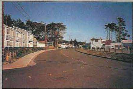
deficient infrastructure elements. As is obvious from the photographs of the finished project, the new Avenue Alhambra does justice to the roadway's prime oceanside location.
