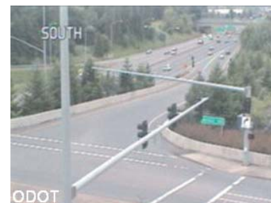
Camera facing the on-ramp at Walker Rd.
