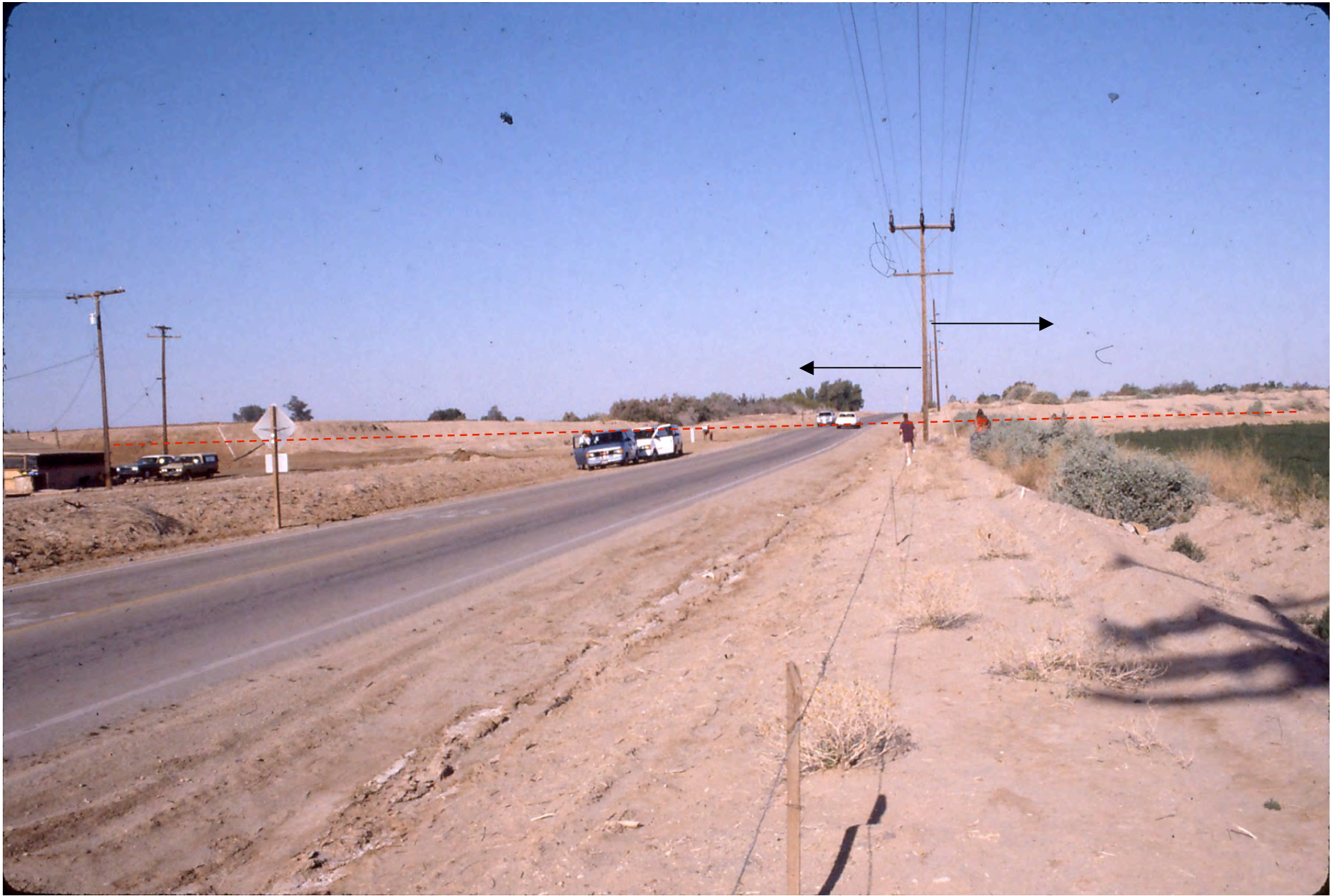
1. Telephone poles showing minor displacement from recent EQ, north of Brawley, CA.
