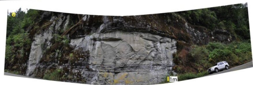
Fig. 6 Unconfined turbidite deposits of central and northern Tye Forearc Basin — proximal and distal deepwater fan deposits;
