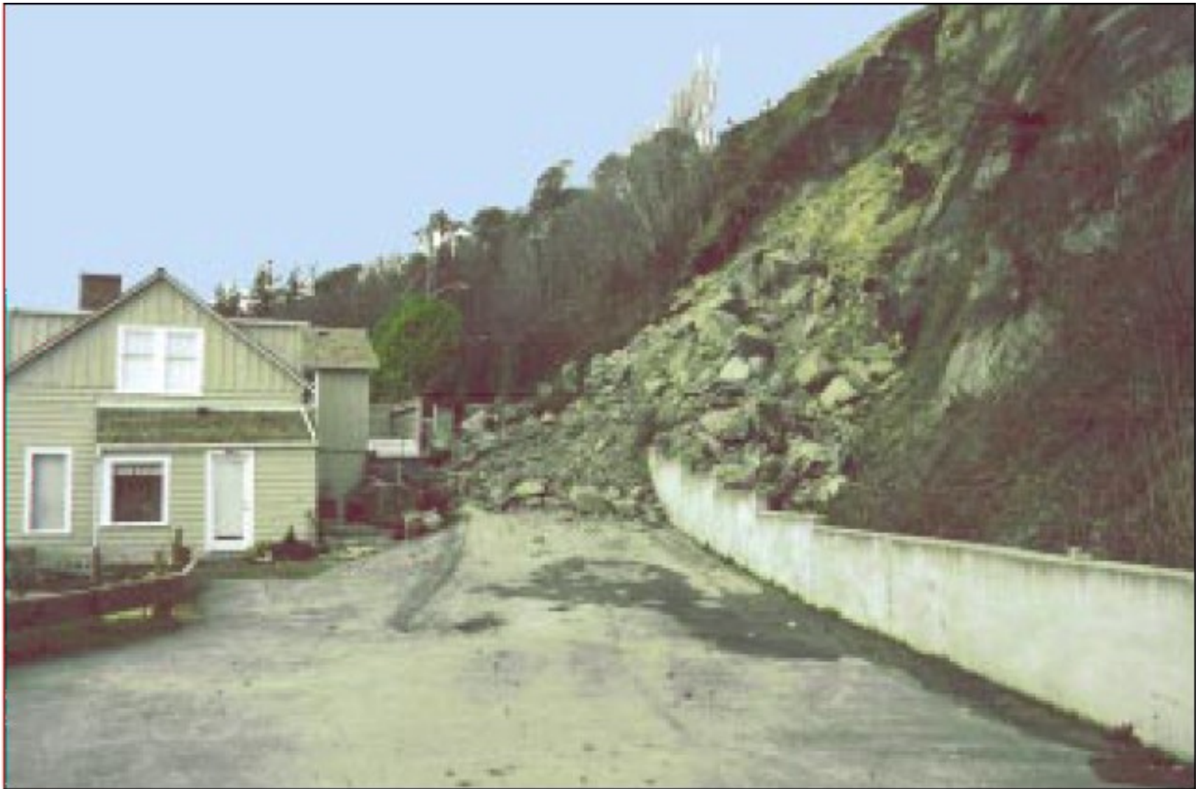
Figure 11. Rock fall next to a house on Perkins Way in northern Seattle. Rock fall is a secondary failure on a larger rotational slump whose failure surface projects beneath the house and Perkins Way.
