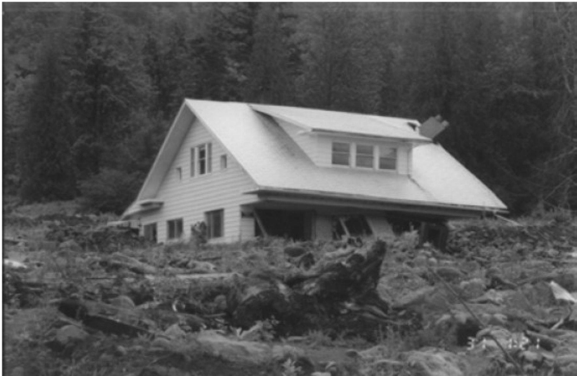
Figure 5. A debris flow destroyed this 2-story residence in Dodson, Oregon in the February 1996 FEMA-OR-1099-OR disaster.
