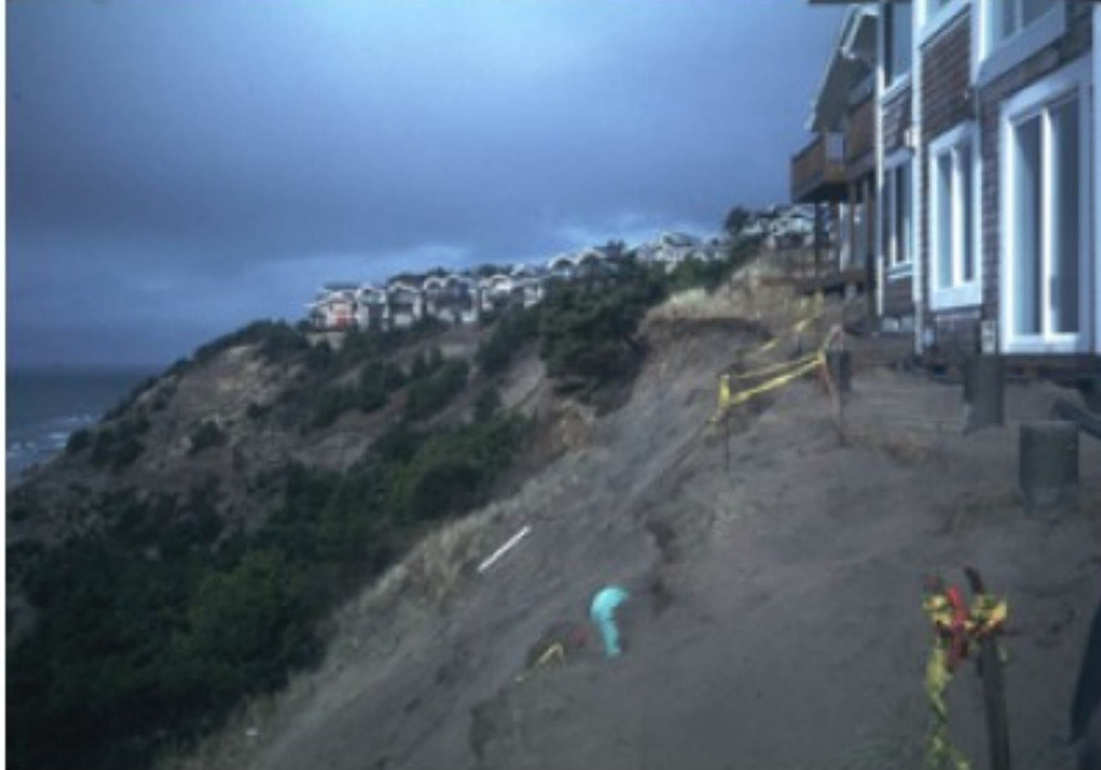
Figure 1. The Capes private housing community experienced landslide and coastal erosion damage associated with the 1997-8 El Nino event. Residents were evacuated and short-term mitigation was implemented. Long-term mitigation options, which need to accommodate coastal building regulations, are still being evaluated. Photo: Paul Komar
