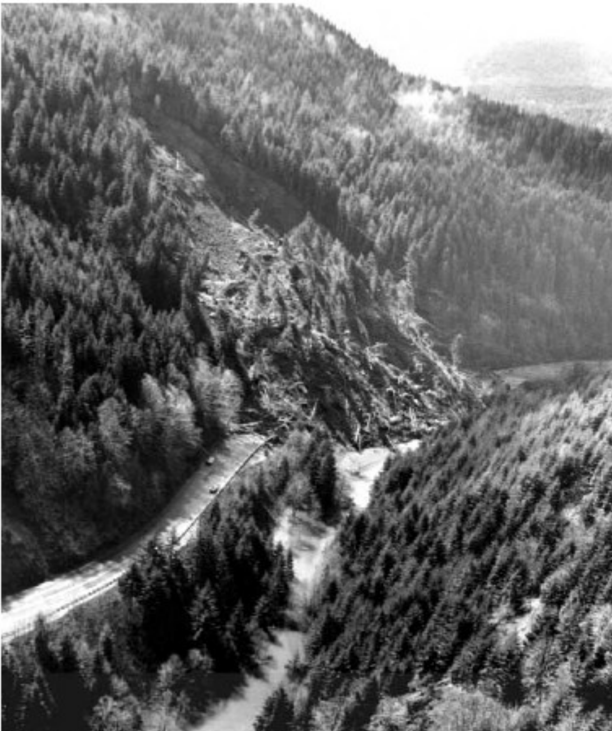
Figure 4. Rockslide that occurred along the Wilson River Highway (Hwy 6) in 1991. Though not a debris flow, this hazardous area is identified by the Further Review Area model. (Photo courtesy of Susanne L. D'Agnesse, Oregon Department of Transportation)
