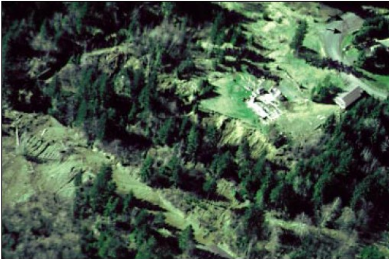
Figure 22. Aerial oblique view of Stevenson landslide. At center right is foundation shown in figure 21. Arrows denote additional extension fractures up-slope from fractures shown in figures 20 and 21.
